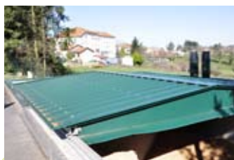
Storeroom for the wood
